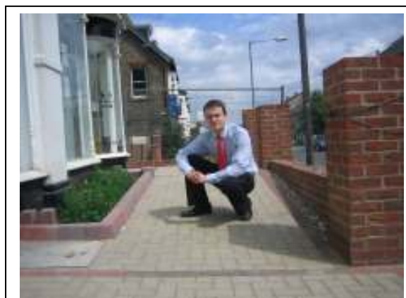
Money wasted on the disabled ramp that was too steep for wheelchair users to climb!
